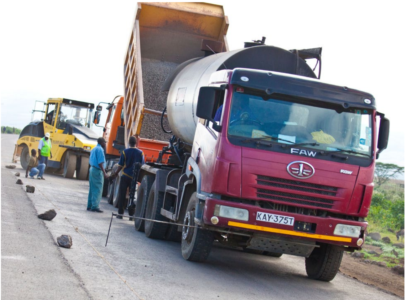
Road construction in rural Kenya
