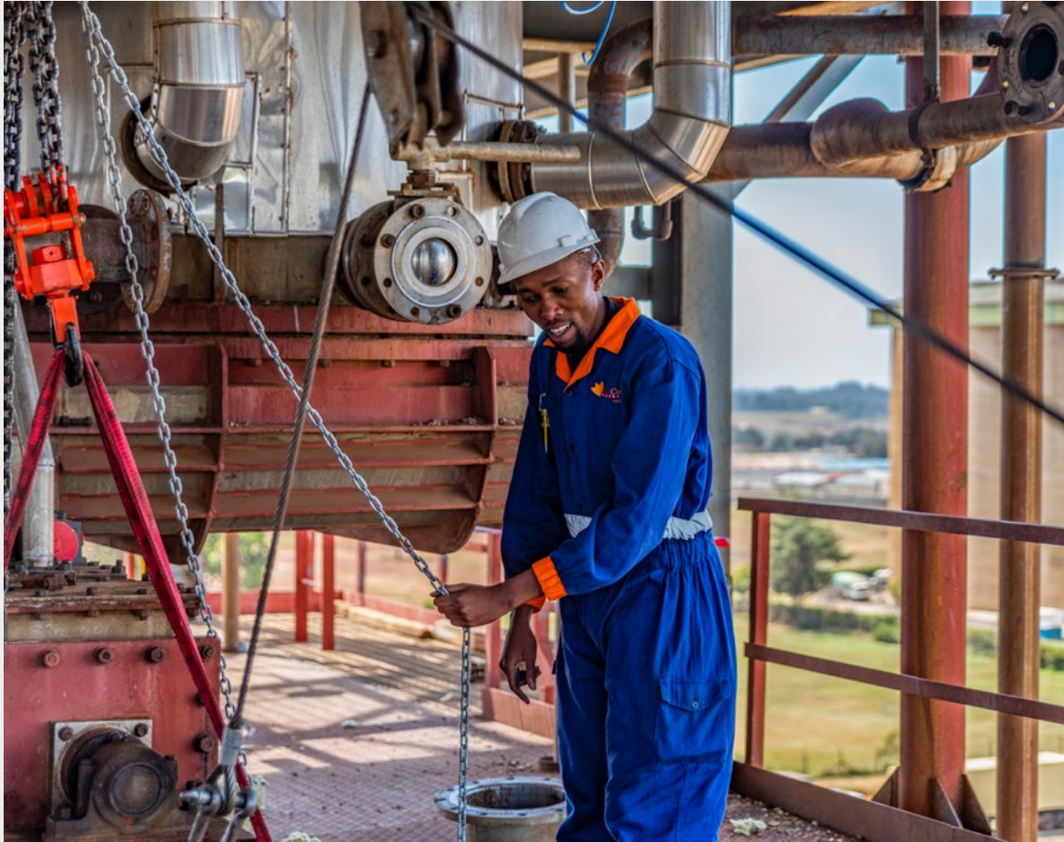
An engineer working on site at a chemical manufacturing plant
